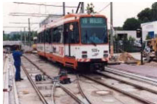
Fig.8 Tram passing over a floating slab
